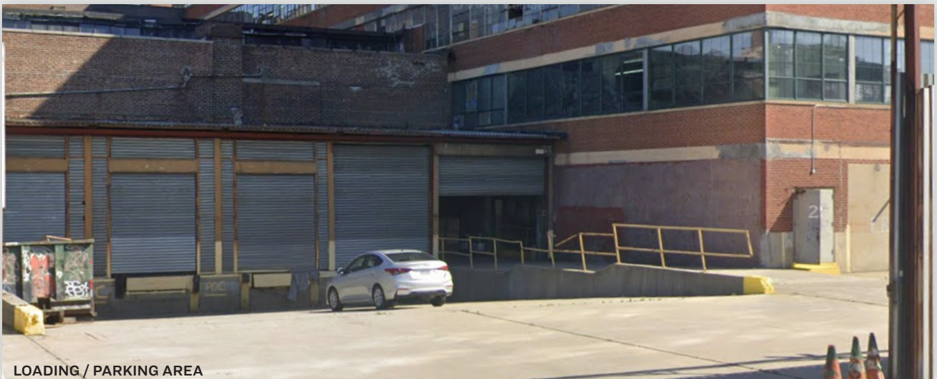
LOADING / PARKING AREA
